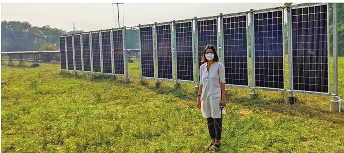
5 kWp pilot site with vertical bifacial modules. © National Institute for Solar Energy (NISE).
