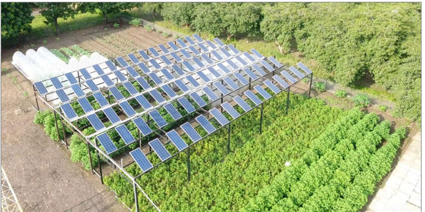
Figure 16: Aerial view of Junagadh agrivoltaic system (Credit: College of Agricultural Engineering and Technology, JAU)
