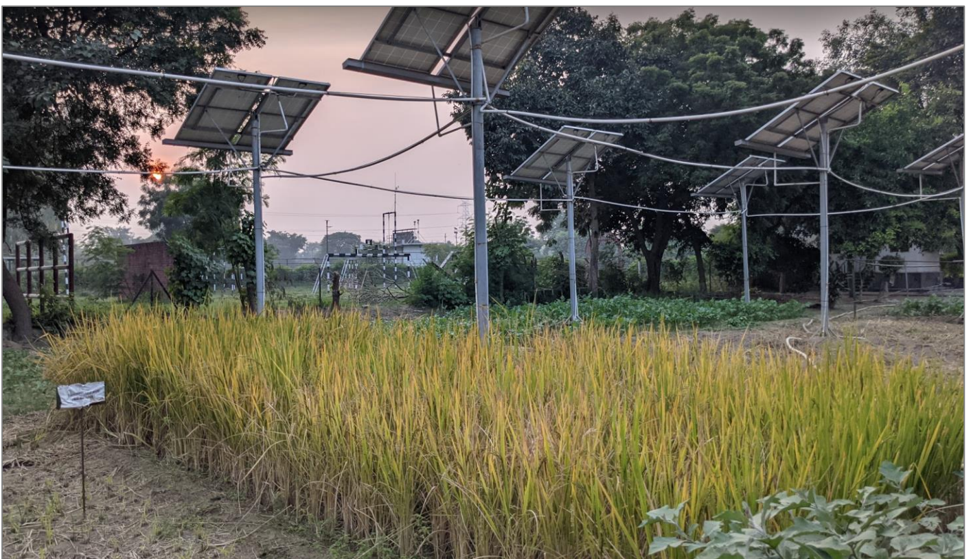
Figure 11: Plant at Amity University (Credit: NSEFI)
