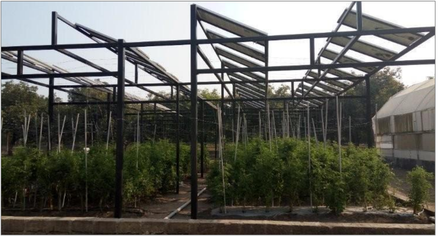
Figure 15: Junagadh agrivoltaic system (Credit: Prof. P.M. Chauhan, JAU)
