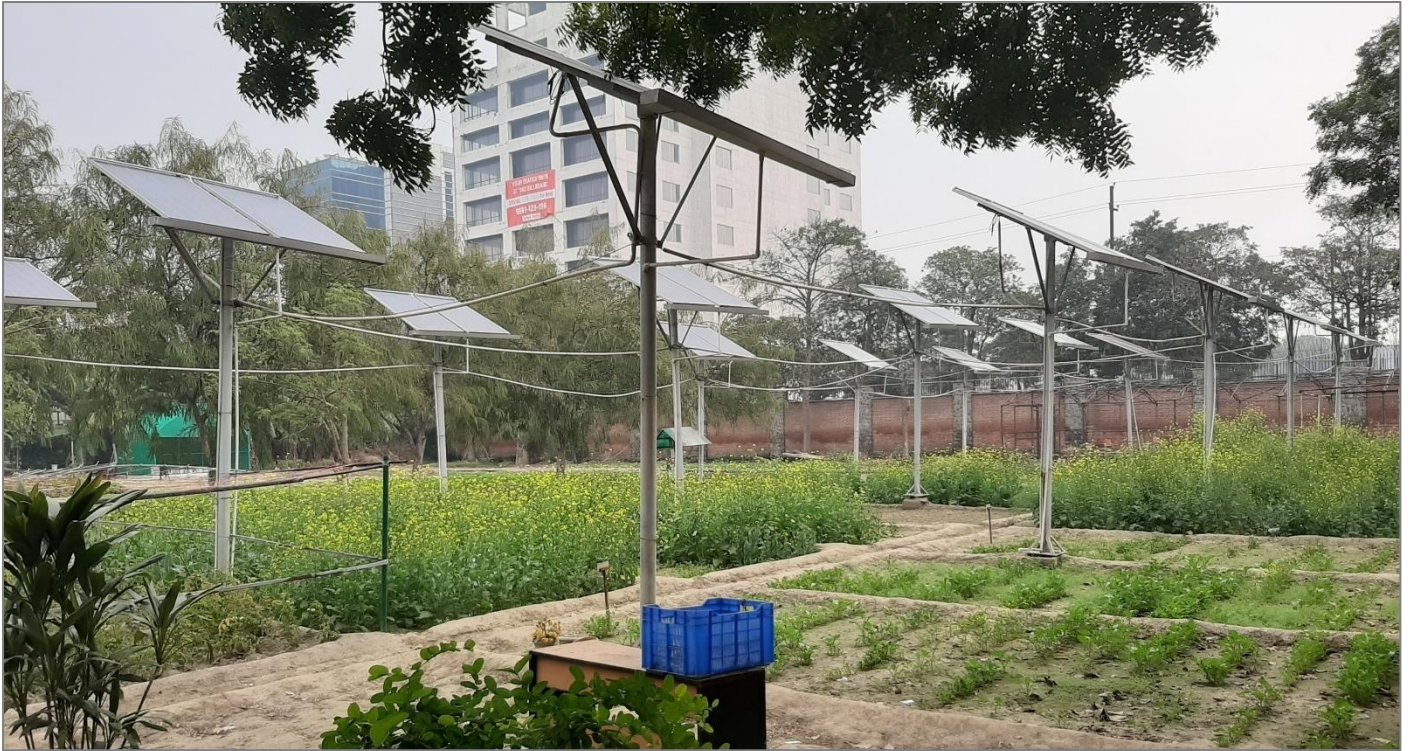
Figure 10: Plant at Amity University (Credit: NSEFI)
