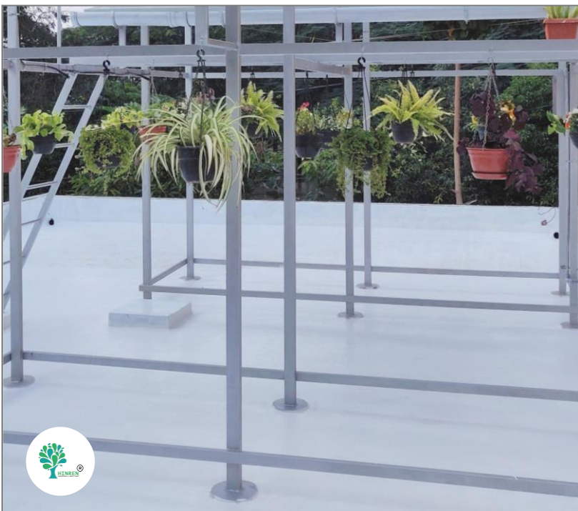
Figure 43: Hinren APVRT structure and white heat seal paint (l), generation profile (r) (Credit: Hinren/Enphase)
