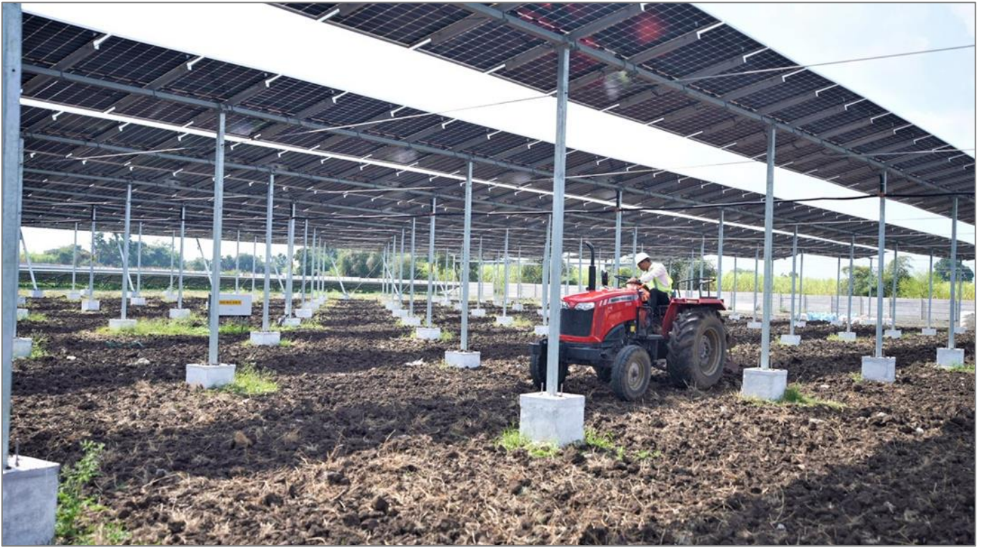
Figure 40: Soil preparation at section I (fully elevated) at agrivoltaics plant near Parbhani (Credit: GIZ)
