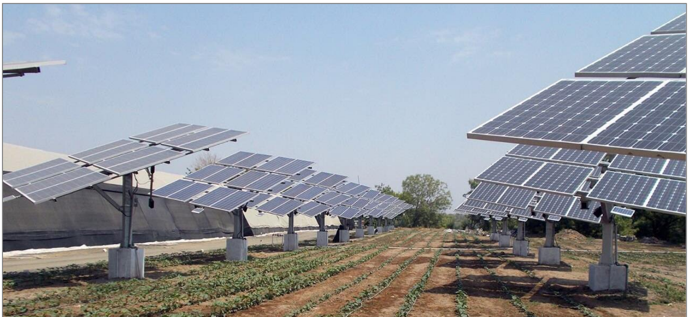
Figure 25: Agrivoltaics with 2-axis tracking and drip irrigation (Credit: Jain Irrigation)
