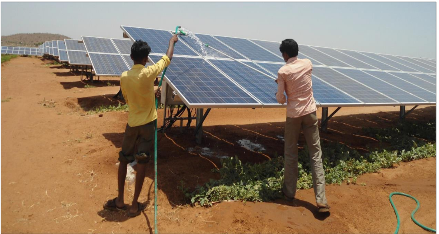
Figure 20: Cleaning and irrigation at Abellon Energy plant (Credit: Abellon Energy)
