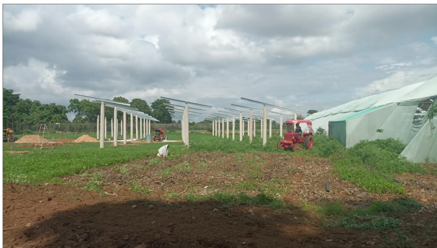
Figure 55: Indra Solar Farm 2 during construction (Credit: Khare Energy Pvt Ltd.)
