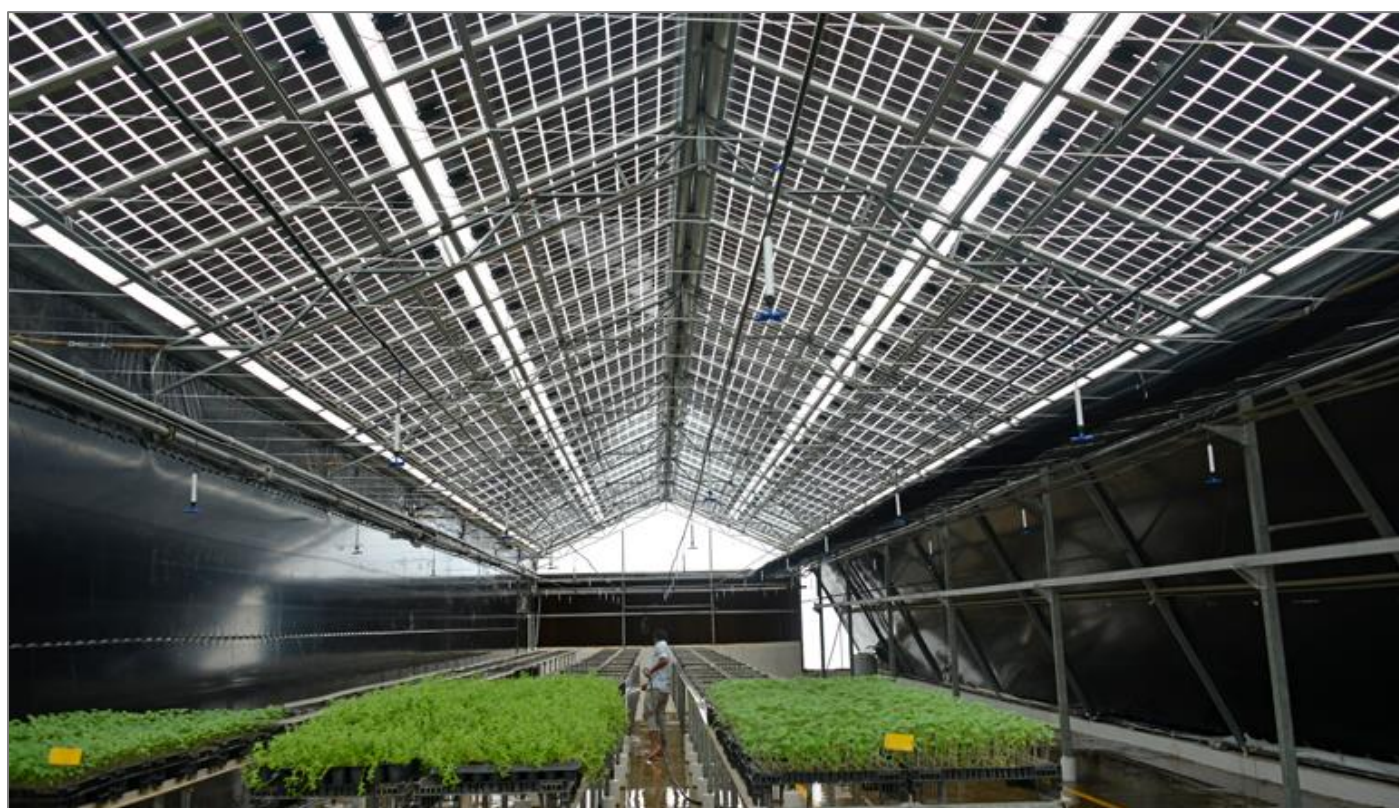
Figure 27: Jain Irrigation Greenhouse PV with Building Integrated Photovoltaic Modules (Credit: Jain Irrigation)
