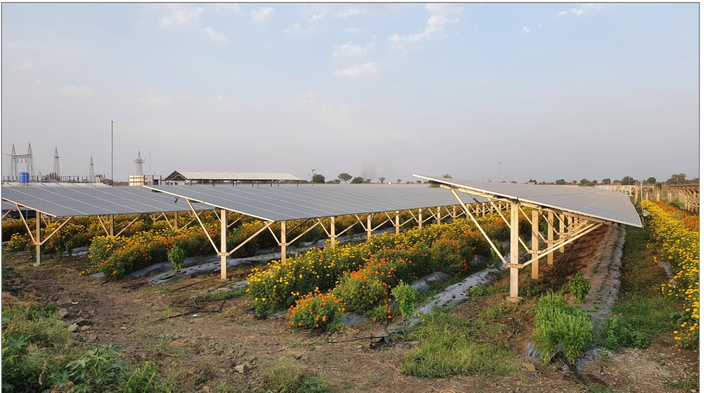
Figure 39: Marigold growing at section II (below and interspace) at agrivoltaics plant near Parbhani (Credit: GIZ)
