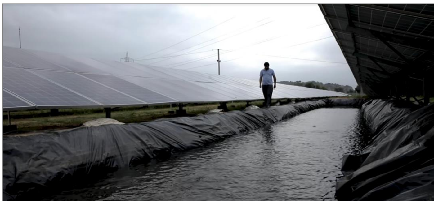
Figure 48: Fish Pond set-up underneath PV-modules (Credit: Down to Earth)
