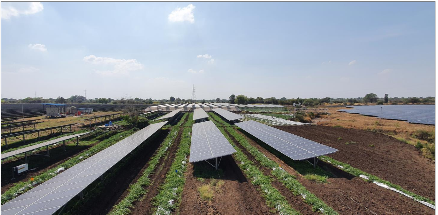
Figure 37: Section IV (Interspace) at Agrivoltaics plant near Parbhani (Credit: GIZ)
