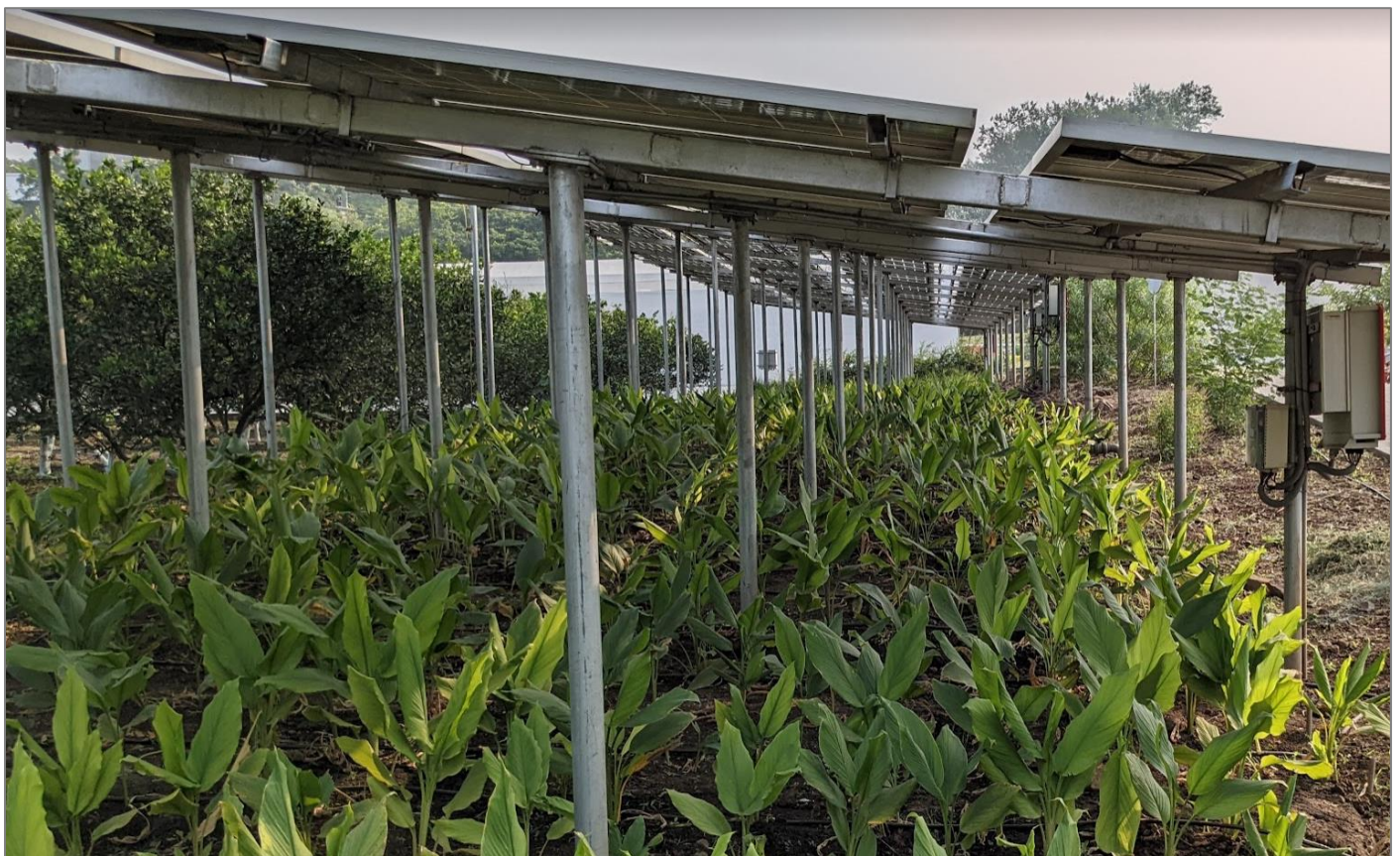
Figure 26: 13.9 kW agrivoltaics system with turmeric (Credit: Jain Irrigation)
