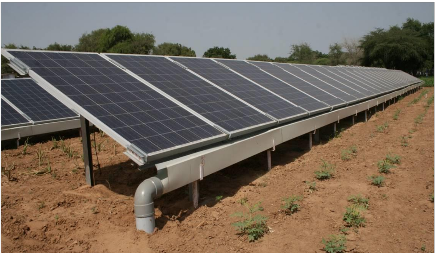
Figure 9: Agrivoltaic system with rain gutter at CAZRI (Credit: CAZRI)
