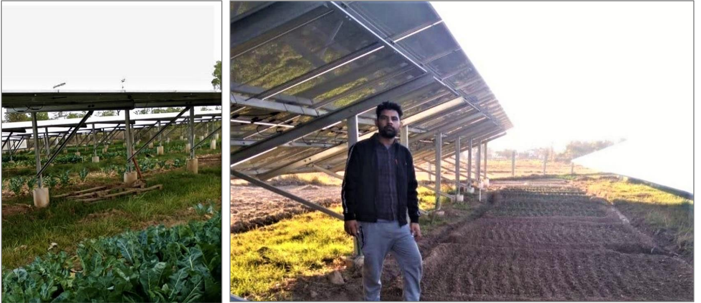
Figure 44: 2.2m elevated Agrivoltaics system near Jahu, Himachal Pradesh (Credit: Gramin Vikas Trust)
