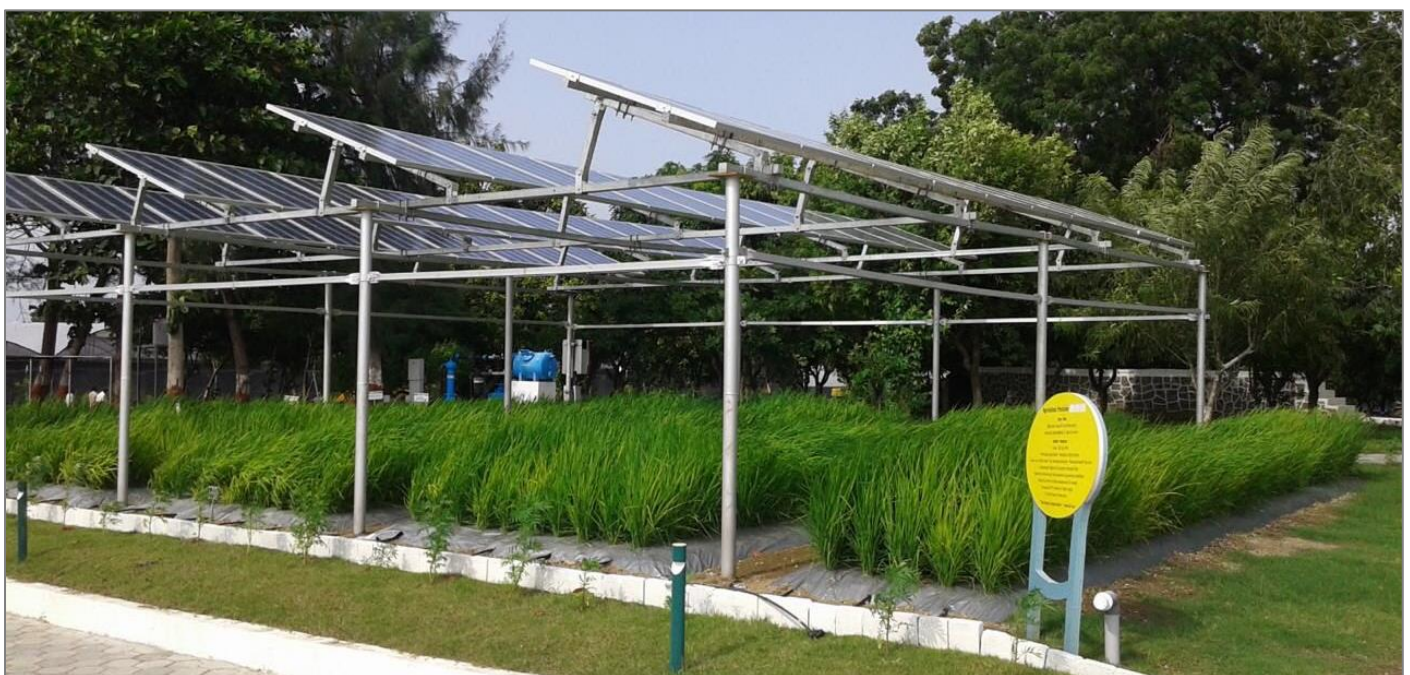
Figure 24: 9.6 kW agrivoltaics system with rice (Credit: Jain Irrigation)
