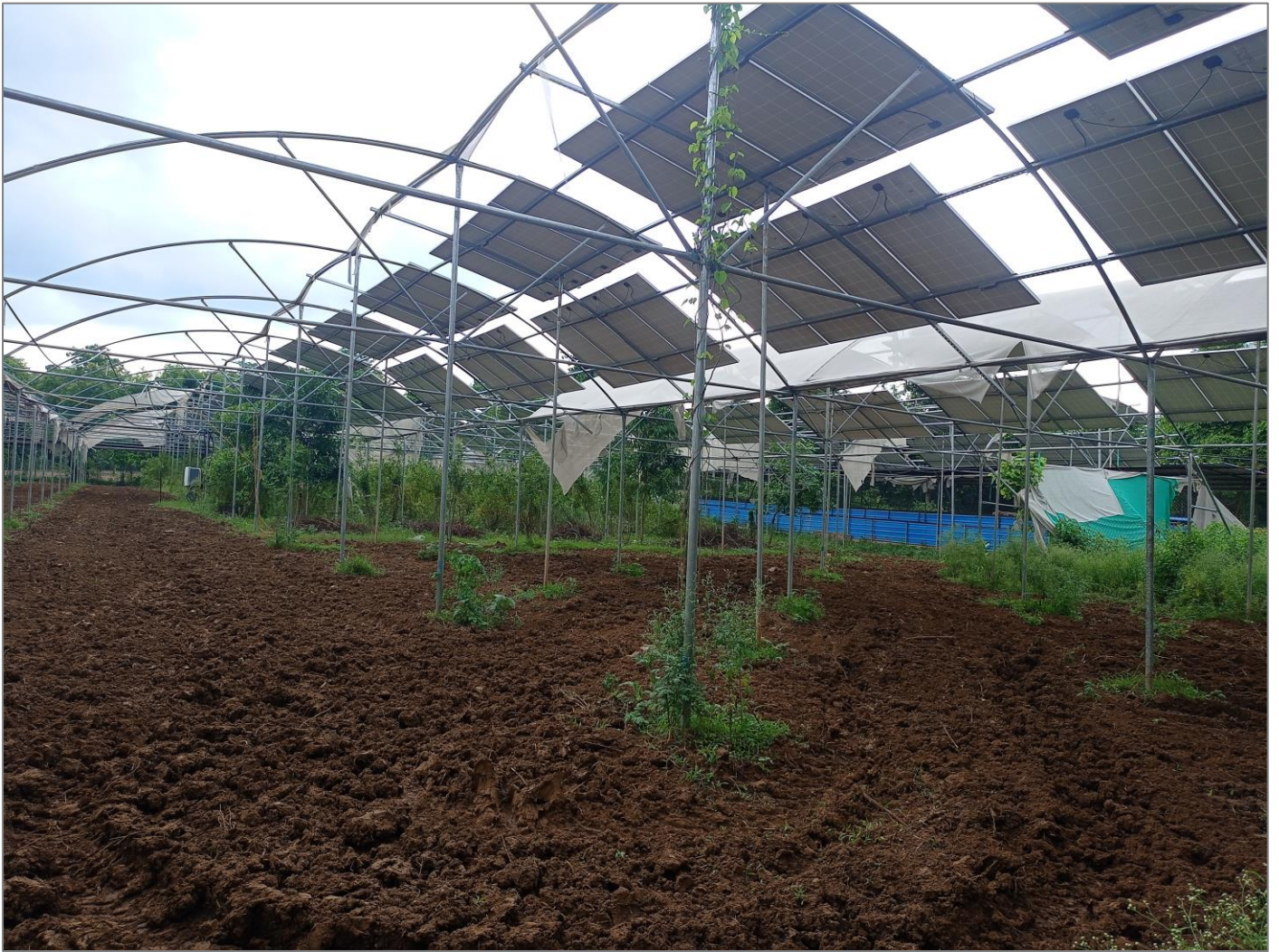
Figure 52: Lightweight polyhouse structure used to mount solar panels at Indra solar farm (Credit: Khare Energy Pvt Ltd.)
