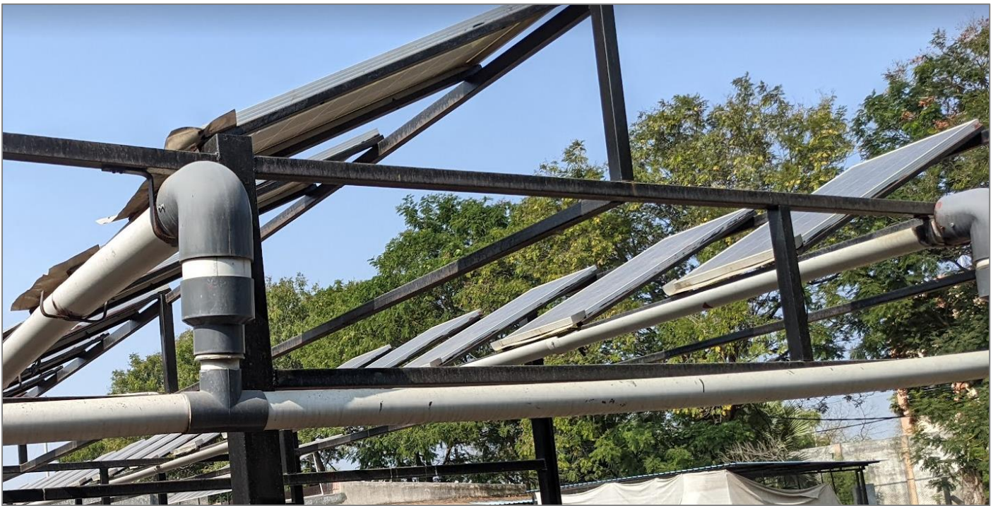
Figure 18: Installed pipe system to collect cleaning water (Credit: JAU)
