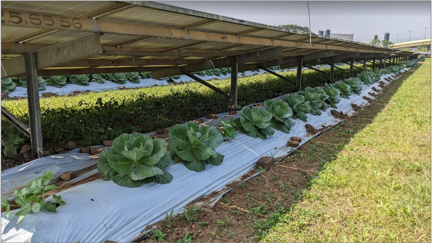
Figure 31: Agrivoltaic plant at Cochin Airport (Credit: CIAL)
