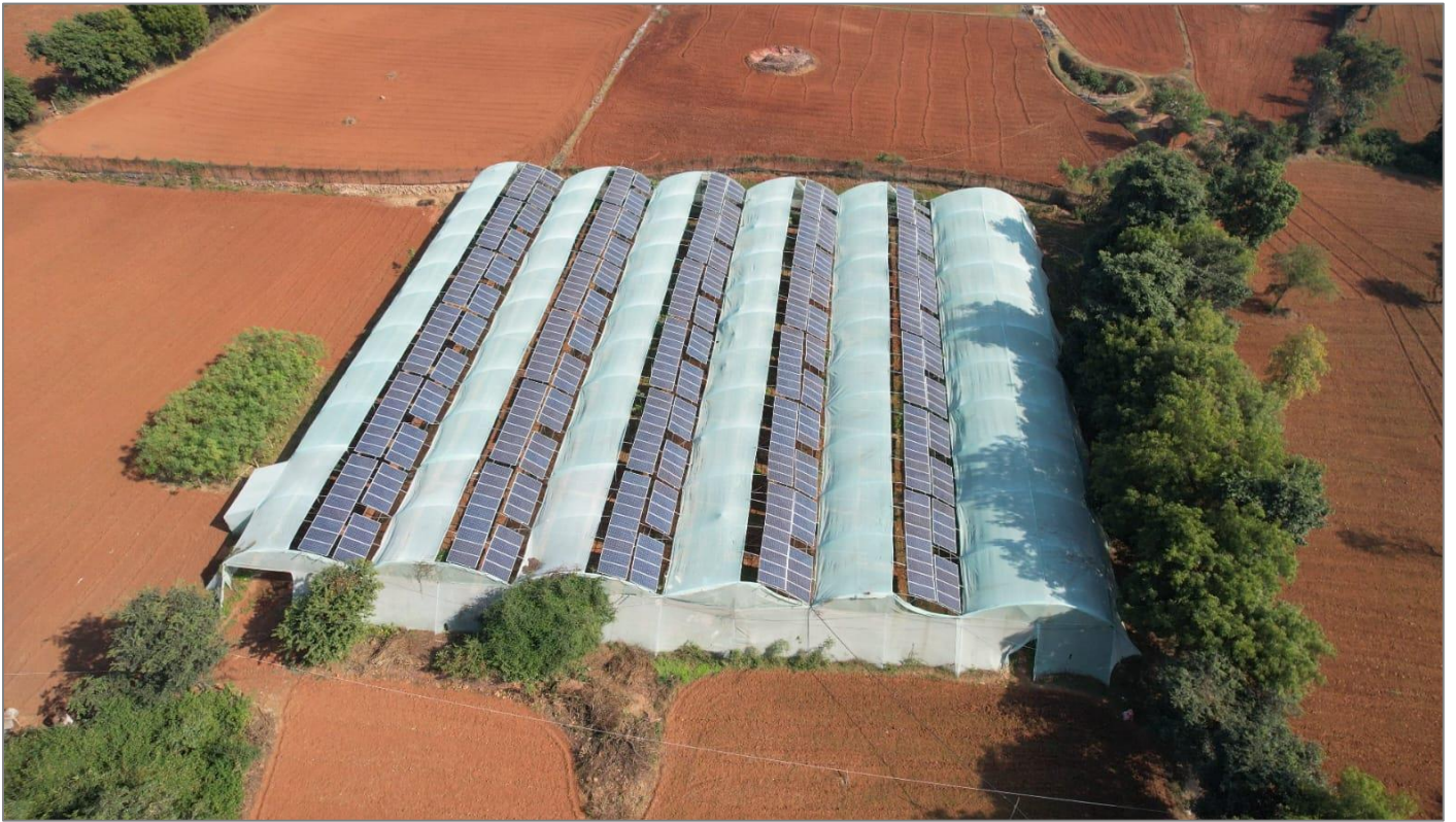
Figure 53: Polyhouse structure at Indra solar farm (Credit: Khare Energy Pvt Ltd.)
