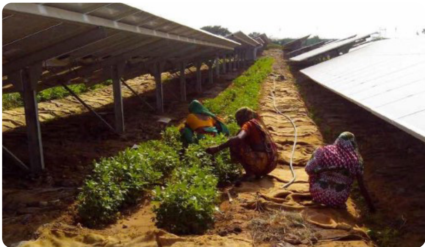
Figure 19: Chilli, 3 MW, Ground-mounted agrivoltaics Site, Gujarat (Abellon)
