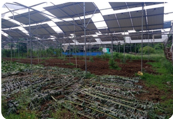
Figure 5: Banana, 1.2 MW, Greenhouse (Khare Energy)
