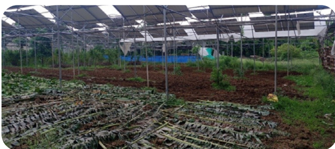
Figure 21: Banana, 1.2 MW, Greenhouse Agrivoltaics System installed by Khare Energy in Madhya Pradesh
