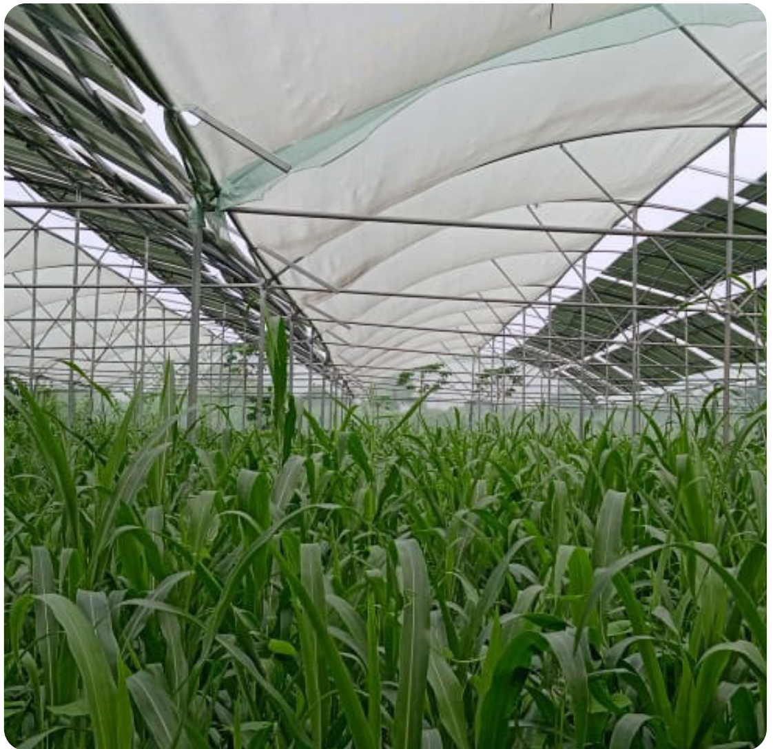
Figure 20: Maize, 1.2 MW, Greenhouse Agrivoltaics Systems, Madhya Pradesh
