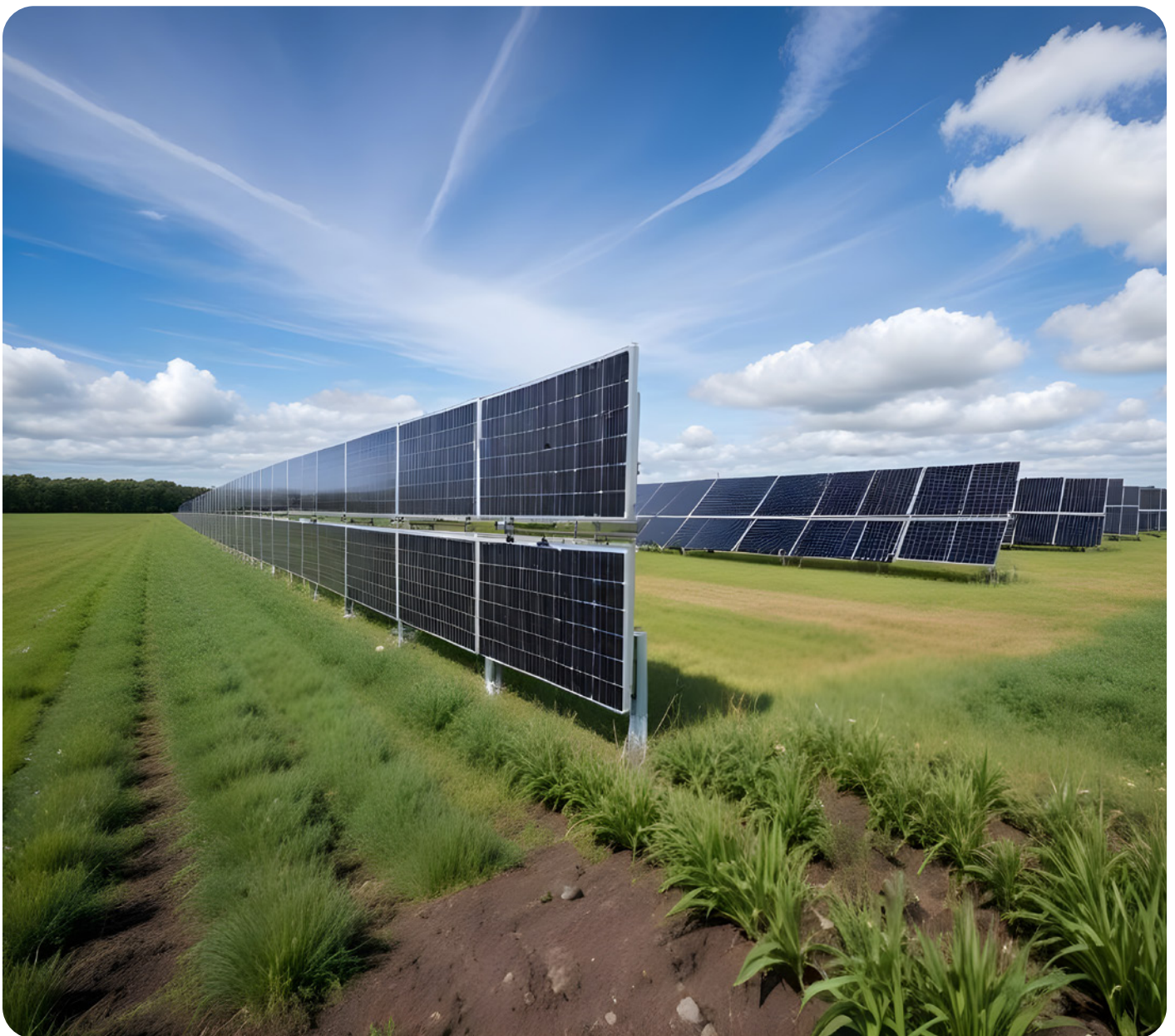
Figure 23: Vertical Agrivoltaics System
