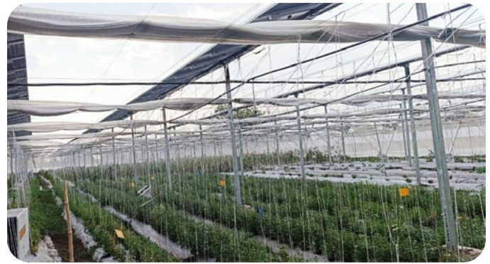
Figure 13: Grapes, 1.4 MW, Sunseed Agrivoltaics site in Maharashtra
